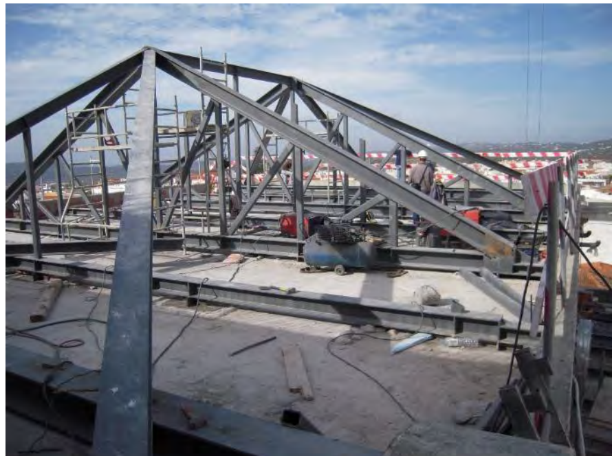
Figure 12_ Roof structure
