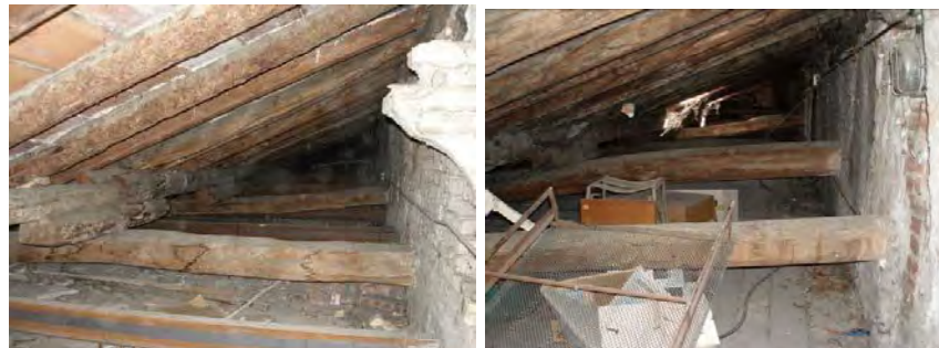
Figure 37_ Internal views of the wooden roof structure
