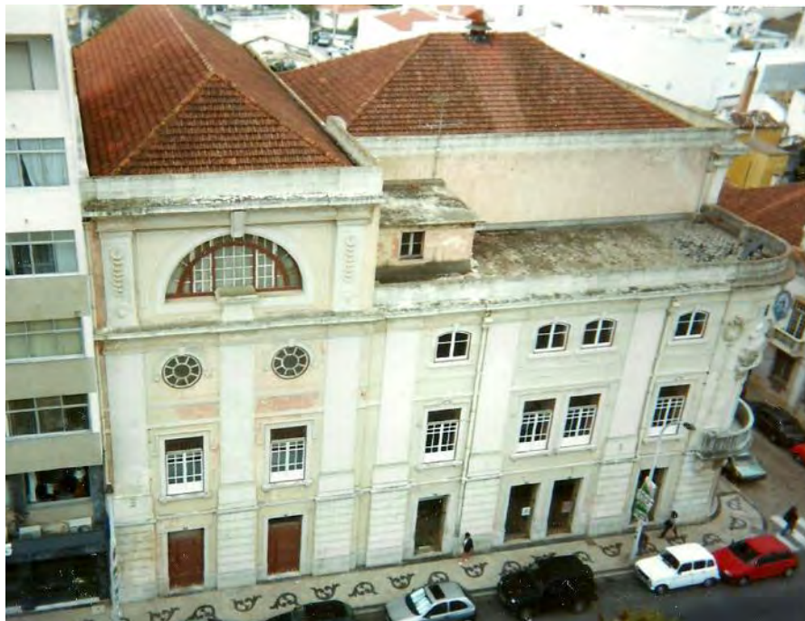
Figure 7_ Aerial view of the state of Cinetatro Louletano before restoration work
