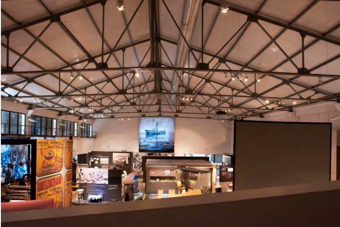
Figure 19_ Temporary exhibition rooms – metal roof
