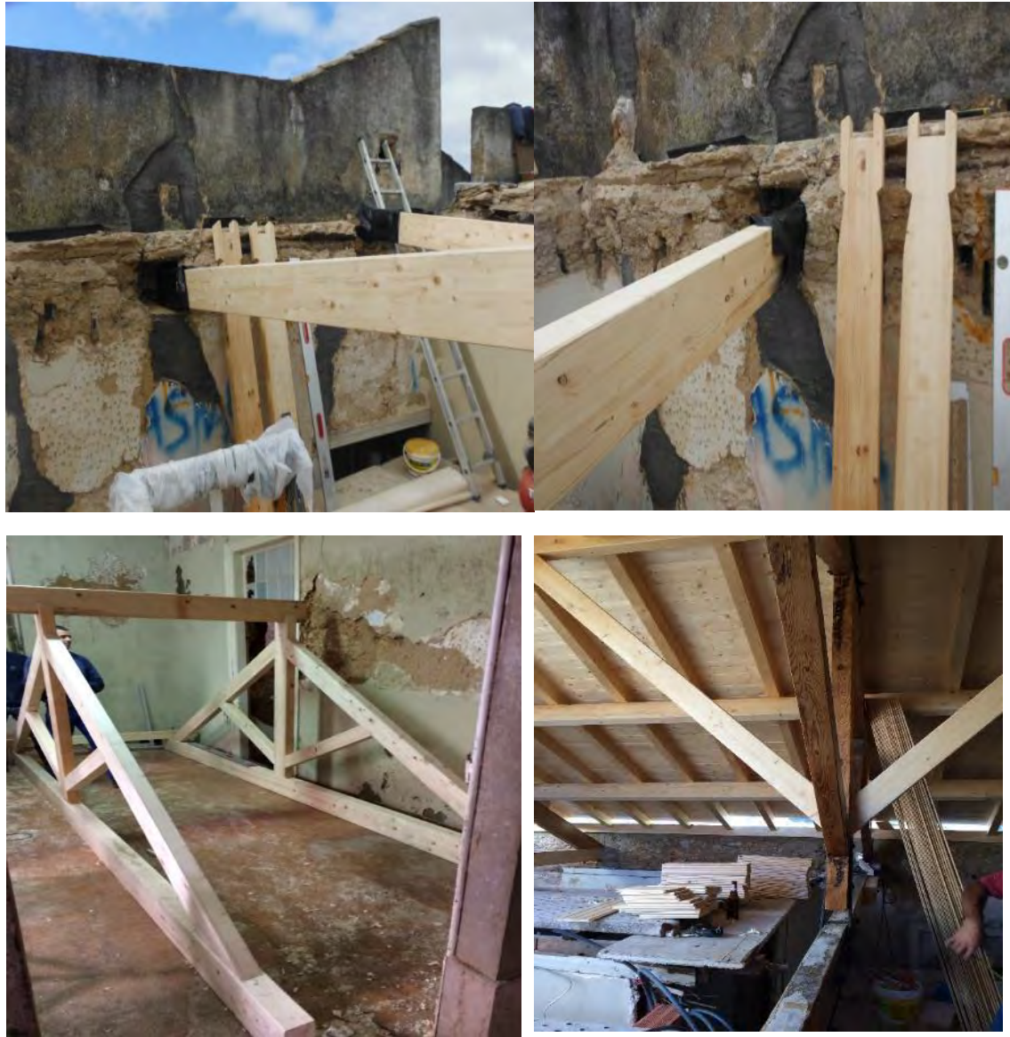
Figure 18_ Intervention in roofs
