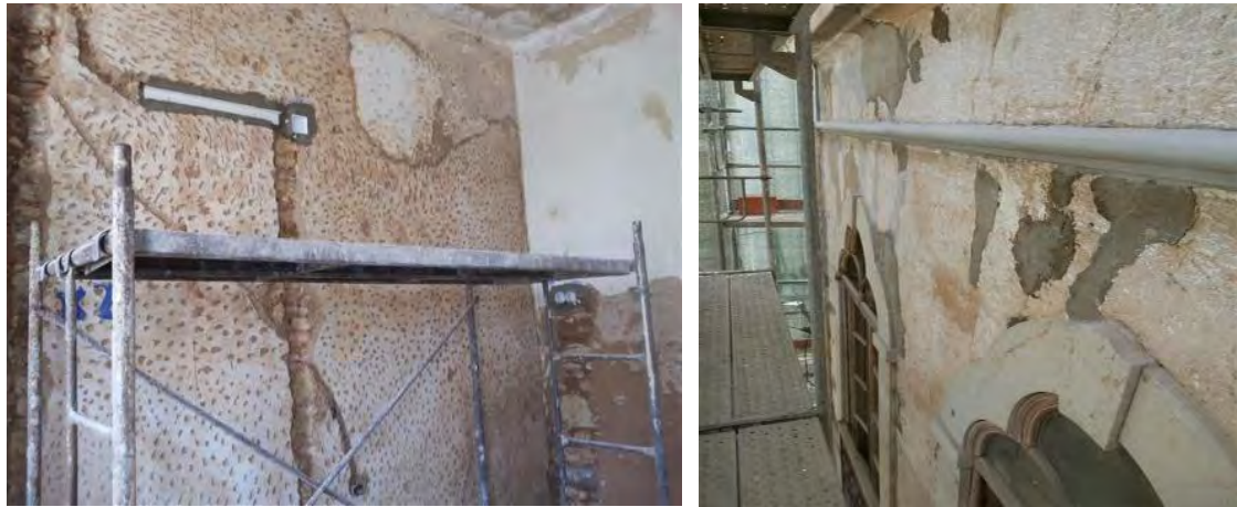
Figure 5_ Walls without plasters.
