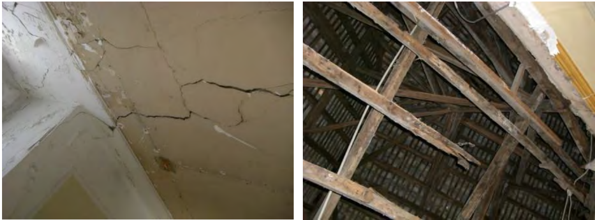
Figure 10_ Pictures of the building (inside) before rehabilitation
