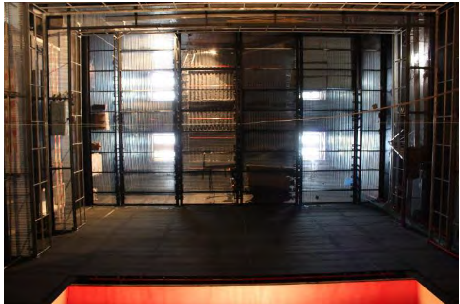
Figure 11_ Assembly phase of the new stage
