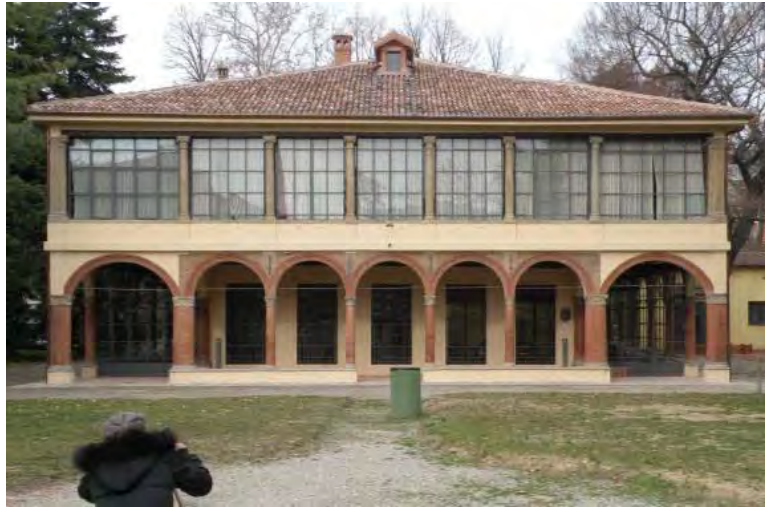
Figure 60_ Main facade after refurbishment work
