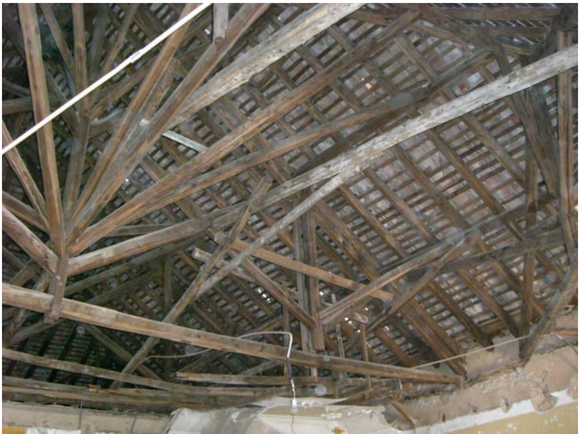
Figure 9_ Picture of the building before rehabilitation
