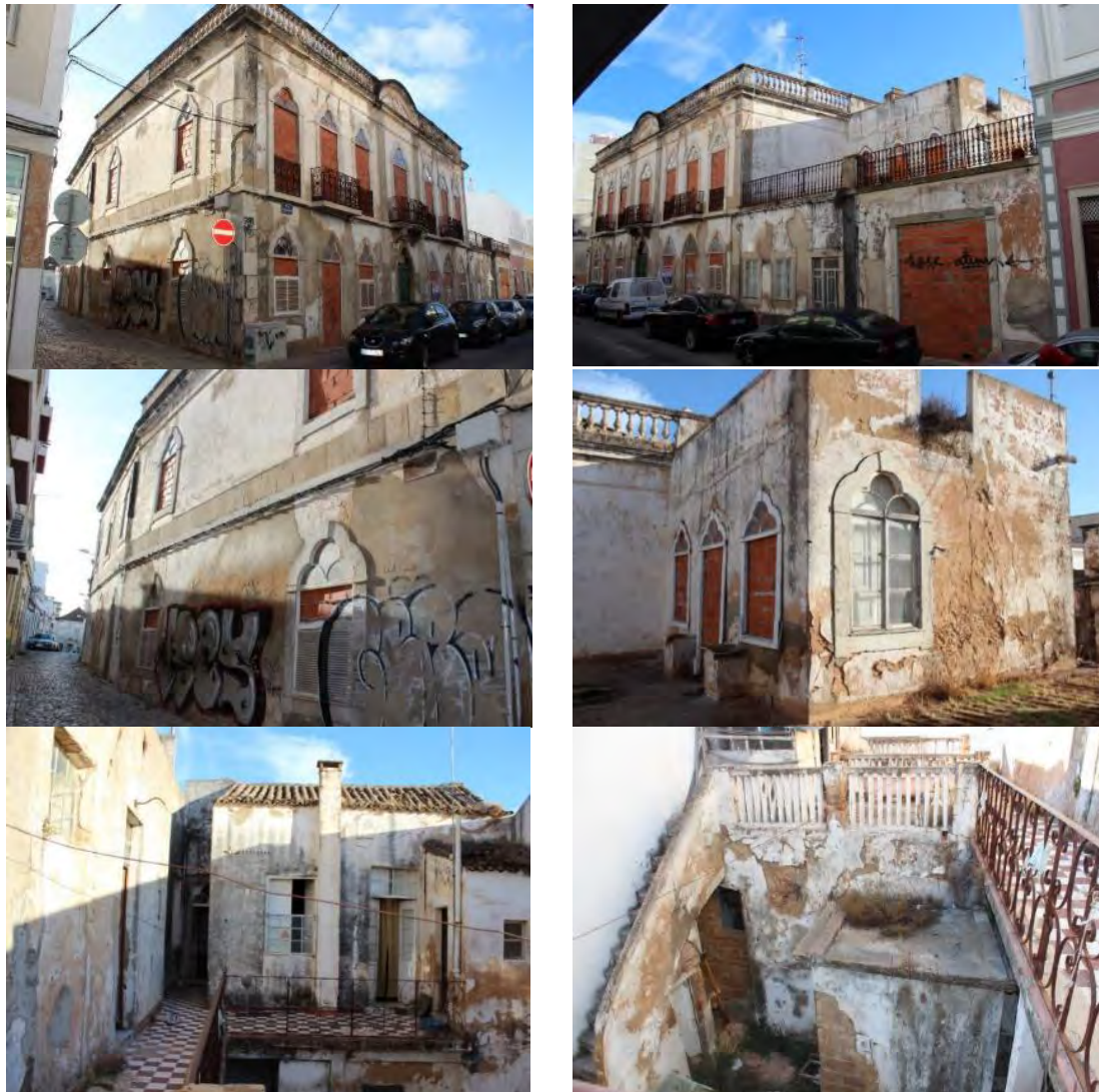
Figure 10_ Pictures of the building before rehabilitation (October 2013)
