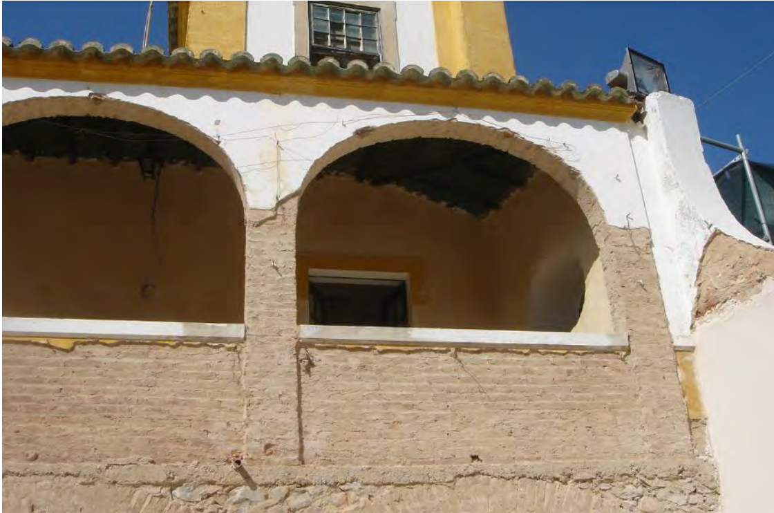
Figure 22_Walls without plasters
