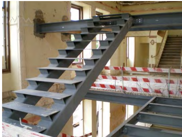
Figure 10_Application of metal stairs from lobby to upper floor (bar).
