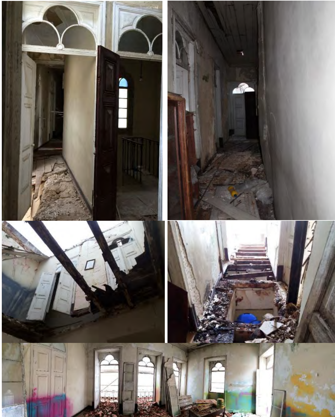
Figure 11_ Pictures, inside the building, before rehabilitation (October 2013)
