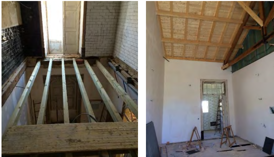
Figure 20_ Reconstruction of floors
