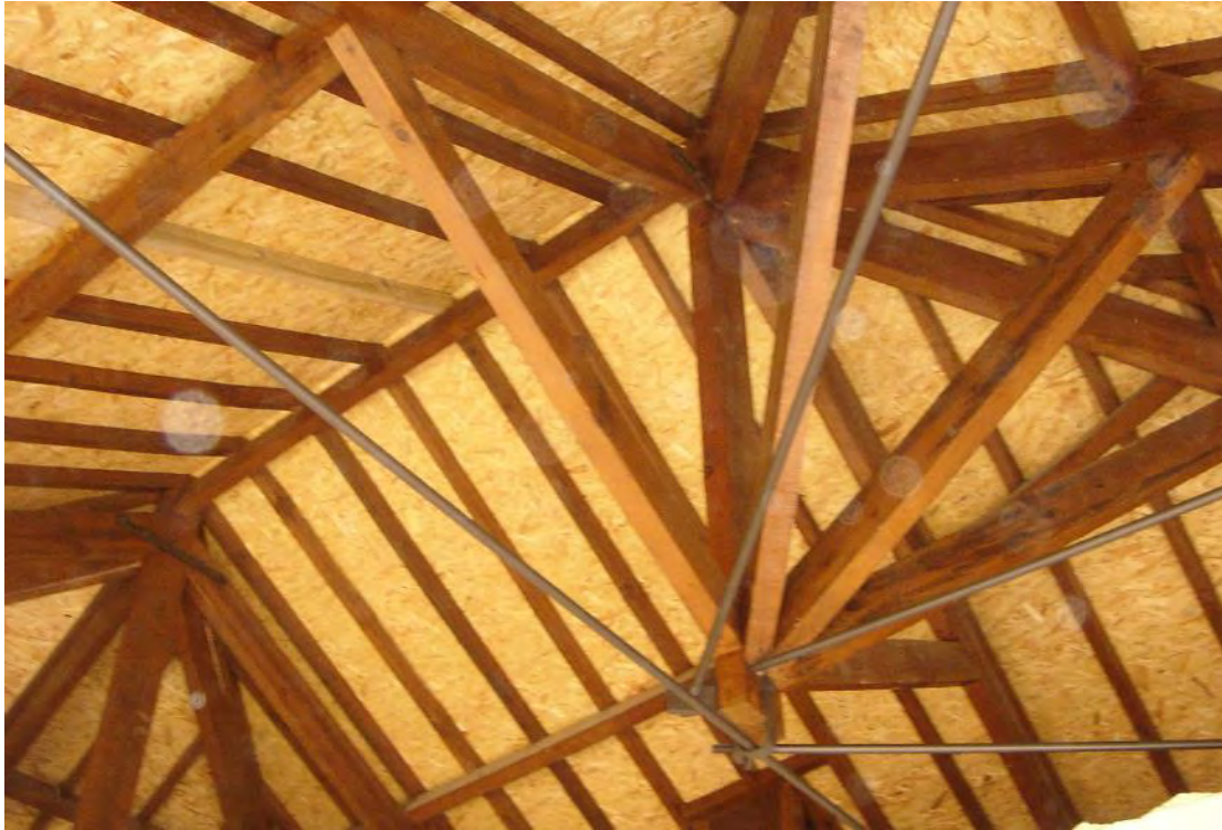
Figure 23_ Intervention in roofs
