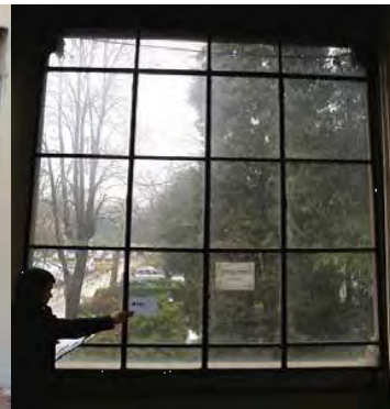
Figure 12_ WIF2, first floor
