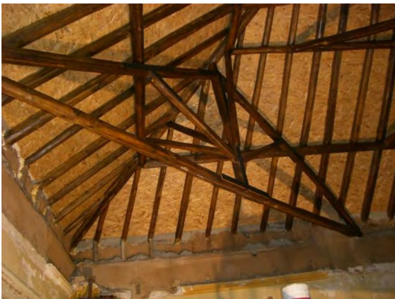
Figure 11_ Rehabilitation of the wood structure of de roofs
