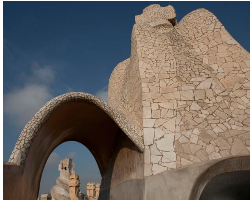
Figure 22: Detail of spiral roof terrace of Casa Milà (Mila House) 70 , Barcelona, with the application of ceramic and marble 71
